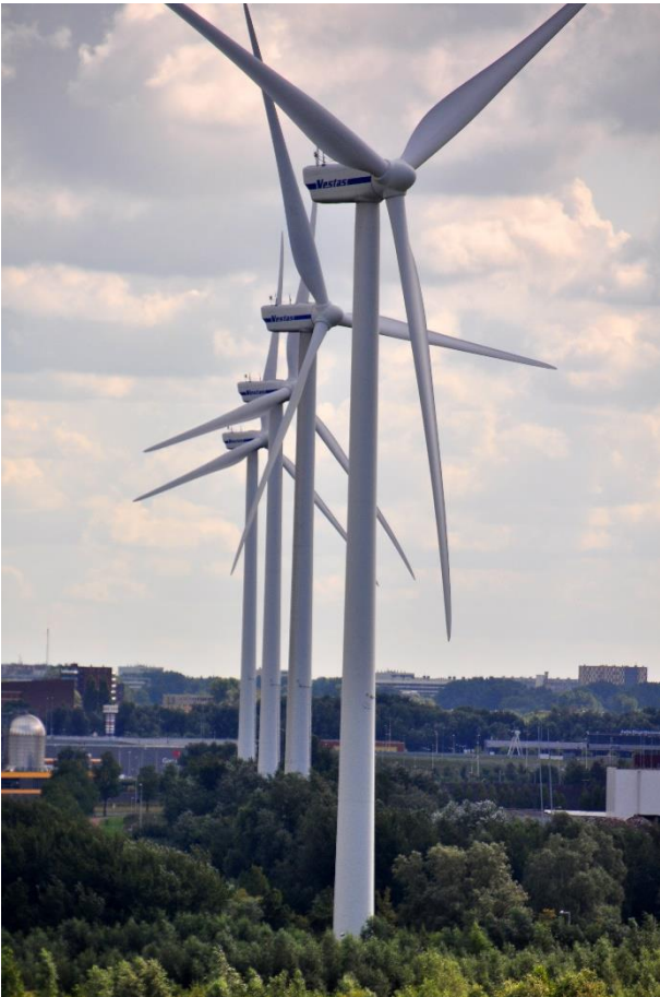
Figure 3. Wind turbine towers
