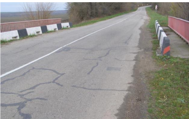
Figure 4: original roadway with kerbs and handrails
