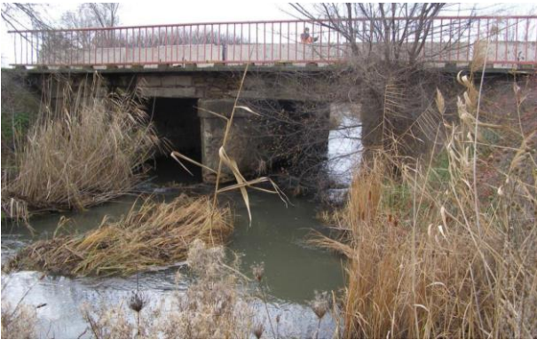
Figure 3: original bridge showing two spans.
