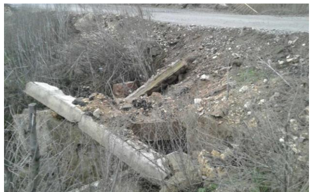
Figure 6: bulldozed temporary crossing.
