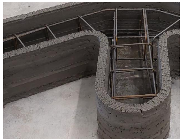
Figure 11: reinforced, 3D printed concrete.
