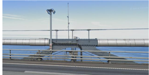
Figure 8. Great Belt Bridge, central clamp
