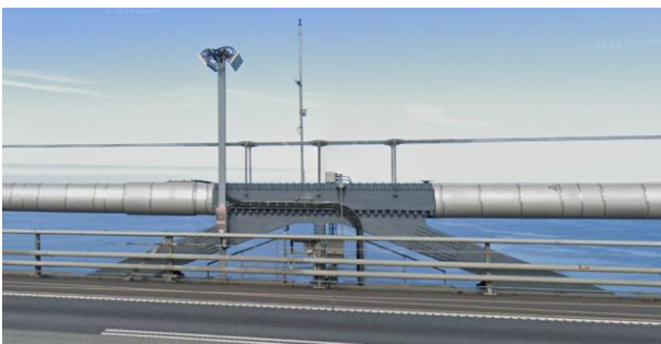
Figure 7. Great Belt Bridge, central clamp
