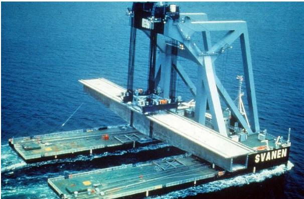
Figure 2. The Great Belt West Bridge, Denmark, under construction [2]
