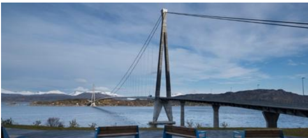
Figure 4. Hålogaland Bridge, Norway (COWI/DW Architecture)
