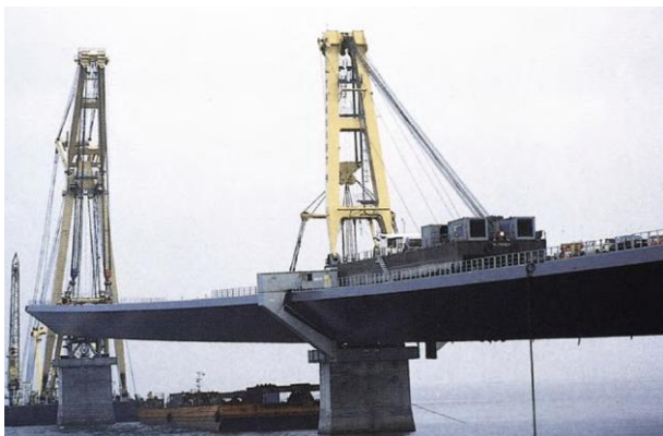
Figure 12. Great Belt East Bridge, placing of span
