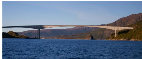
Figure 8. Raftsundet Bridge, Norway [6] (photo: broer.no)
