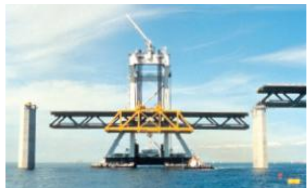
Figure 14. Erection of Øresund Bridge viaduct span
